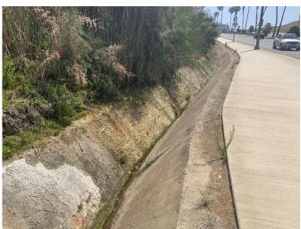
Photo 8: Superior Avenue wetlands. Note excess water draining off slope into the concrete-lined drainage ditch at toe of slope.
